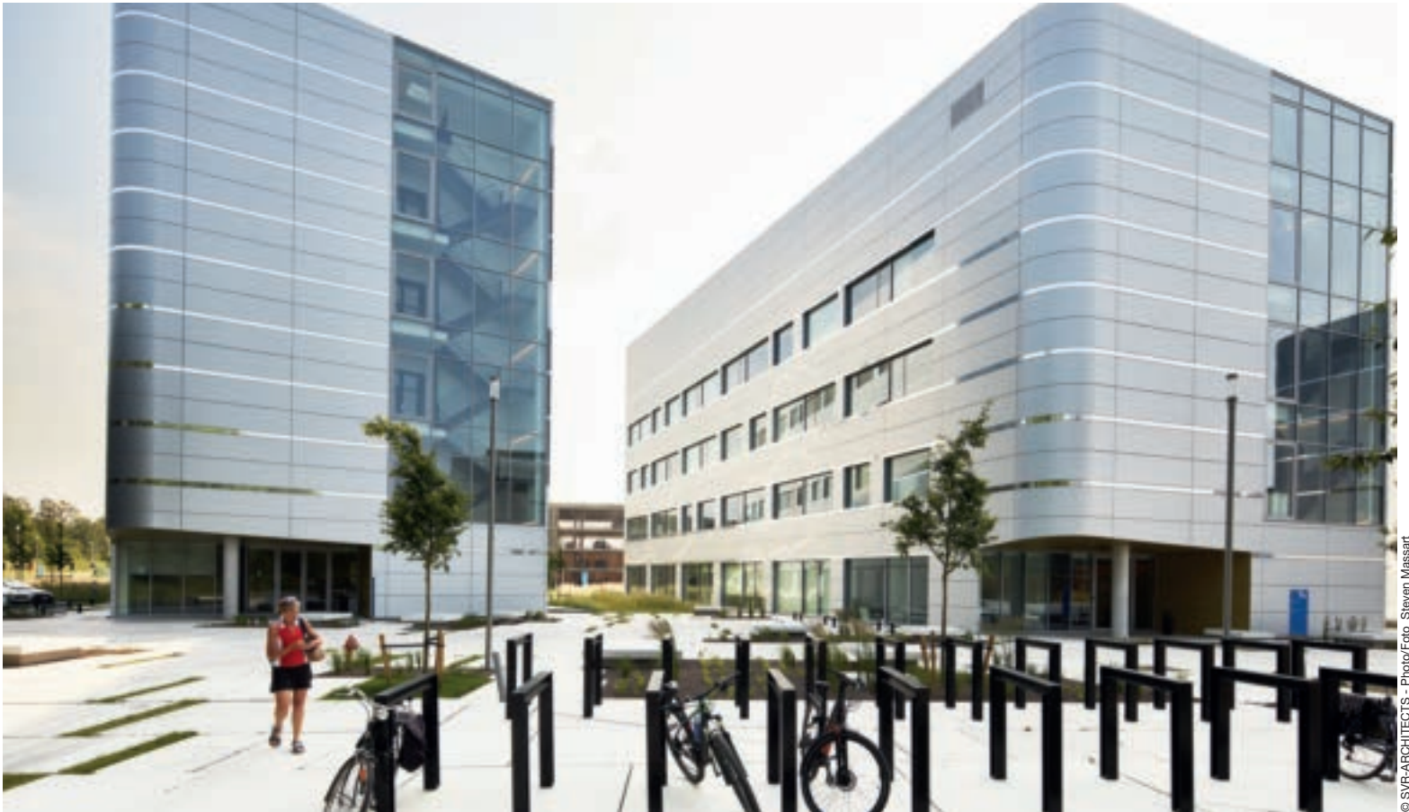
© SVR-ARCHITECTS - Photo/Foto Steven Massart
