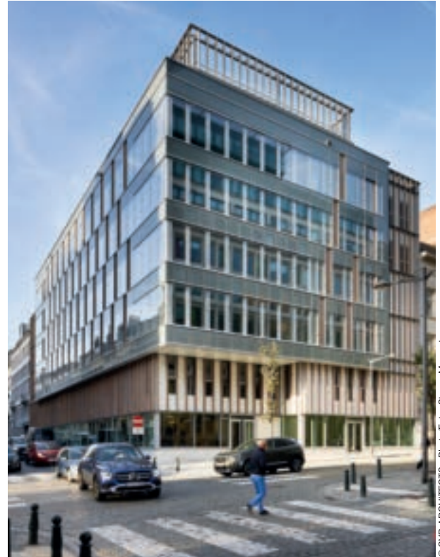
© SVR-ARCHITECTS - Photo/Foto Steven Massart
